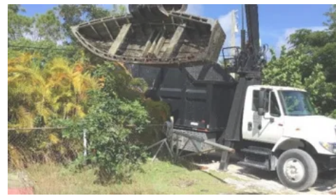
Public Invited to Celebrate Clearing of Last Irma Canal in NRCS Marine Debris Removal Project - ThursdayJo October 22, 2019
